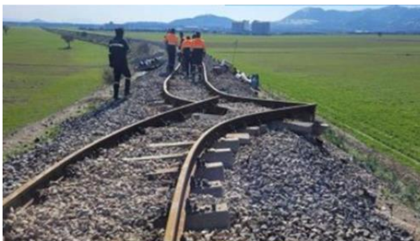
Figure 2. Deformations in Fevzipaşa railway (KG, 2024)
